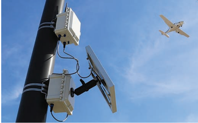
Pole-mounted Version II device installed at Terre Haute Regional Airport (KHUF) for data collection at a towered airport.
