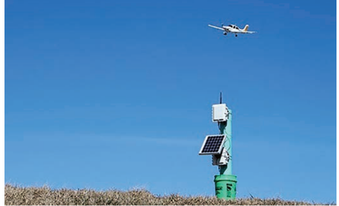
Stand-alone Version II device installed at Indianapolis Executive Airport (KTYQ) for data collection at a non-towered airport.
