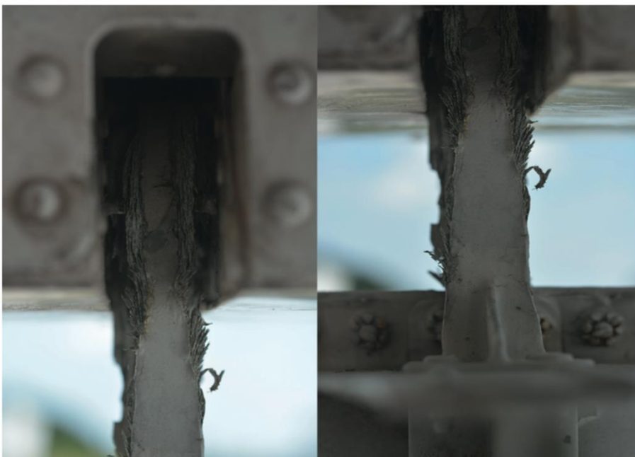
To expertise is to explain effects, in this case those of corrosion.
